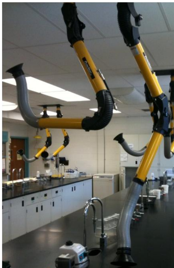
Fig. 13 Elephant Trunks in Essex Hall Undergraduate Labs
