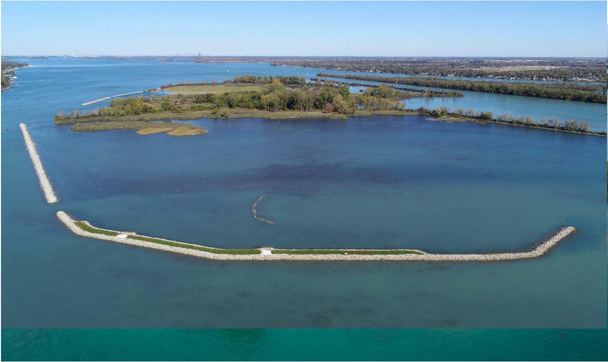
Figure 1. A new habitat shoal off the south shore of Stony Island protects a fragile coastal wetland from further erosion and creates over 20 ha of calm backwater for fish spawning and nursery (credit: Friends of the Detroit River).
