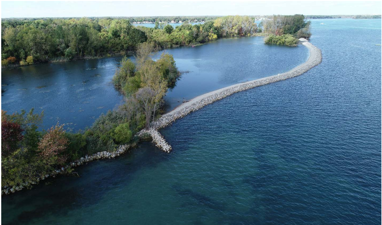
Figure 3. A new habitat shoal protects fragile coastal wetlands at Celeron Island's north bay from further erosion and enhances this backwater area for fish spawning and nursery activity (credit: Friends of the Detroit River).
