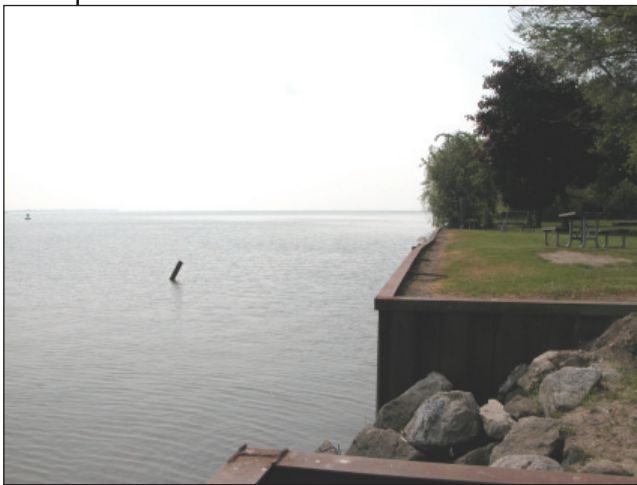
Figure 1. Lake Erie shoreline hardening with steel sheet piling (Photo credit: Greg Norwood).
