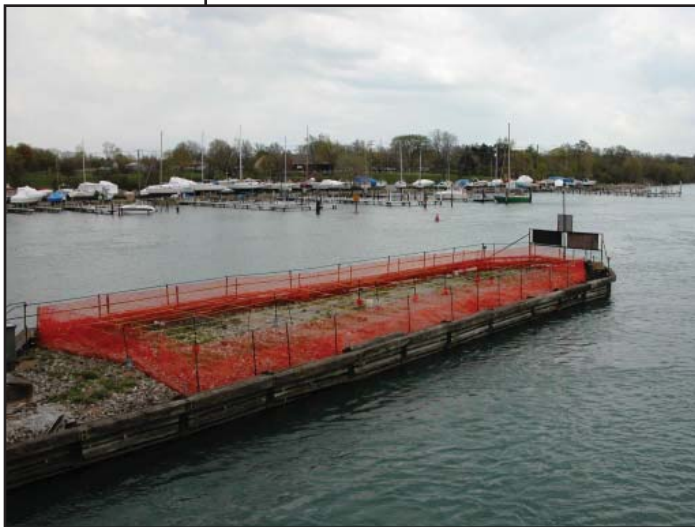
Figure 1. The rope-lattice structure of one side of the swing bridge used to deter black-crowned night heron predation.
