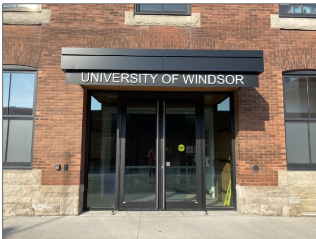
2 West entrance to Armouries, facing Freedom Way.
