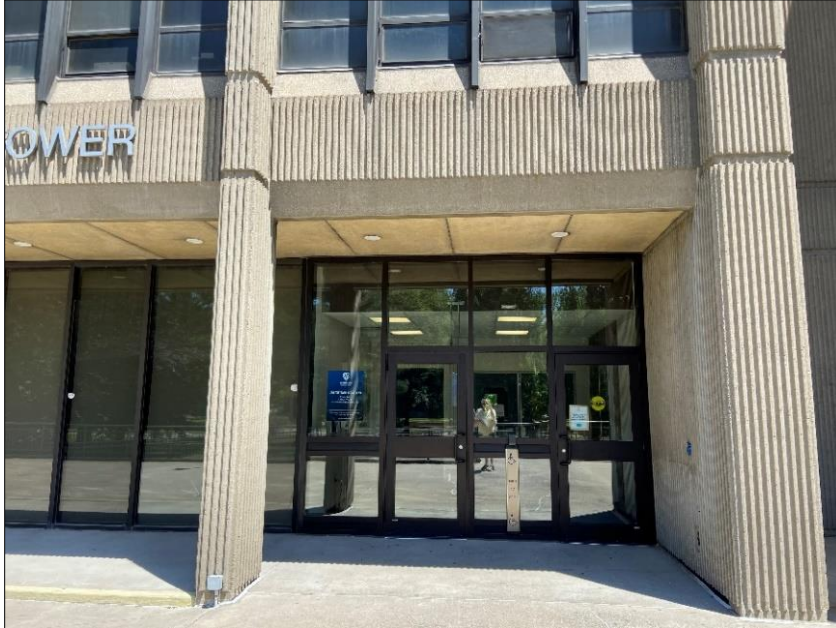
The west accessible entrance to Lambton Tower
