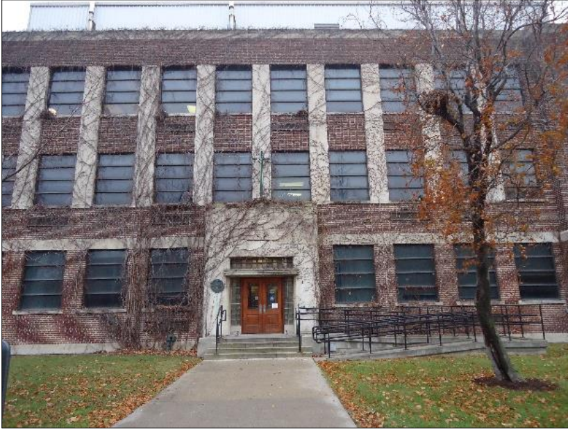
Exterior view of Memorial Hall
