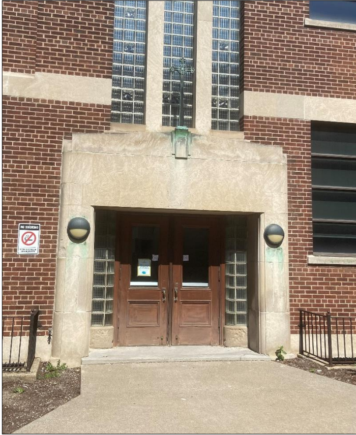
Additional entrance on the northeast corner. It is ground level with no actuator.
