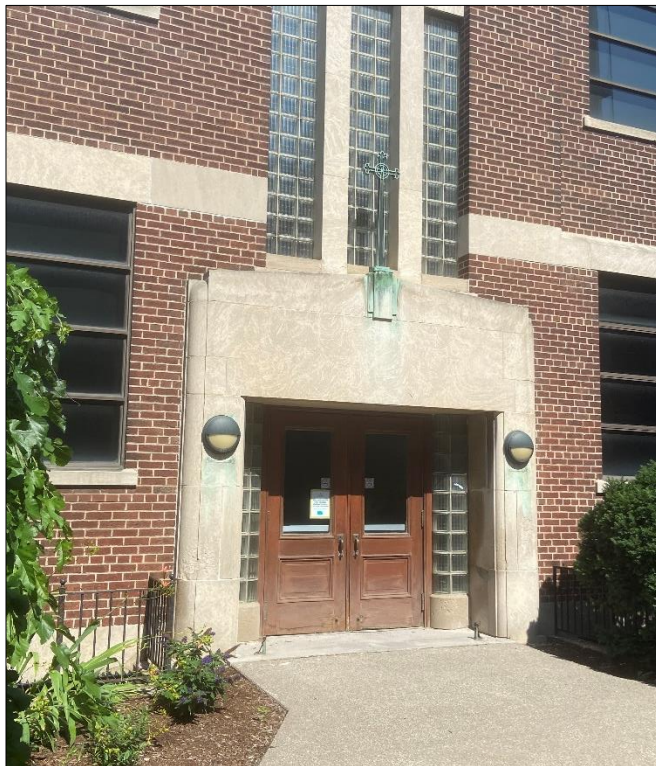
Additional entrance on the northwest corner. It is ground level with no actuator.
