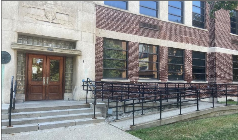
Main entrance of Memorial Hall, equipped with a ramp and actuator.
