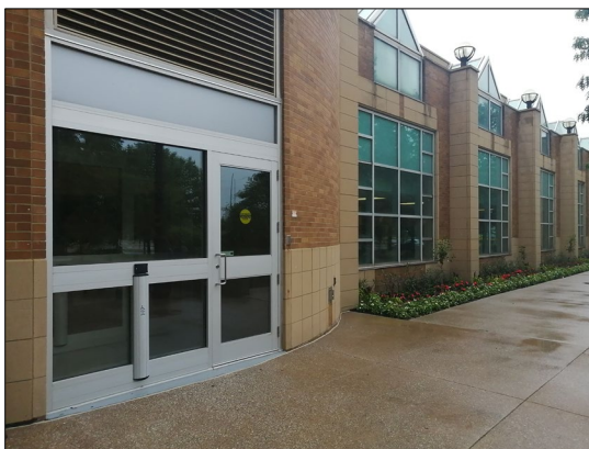
Accessible Entrance to East Wing of Odette School of Business
