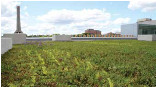
The green roof
